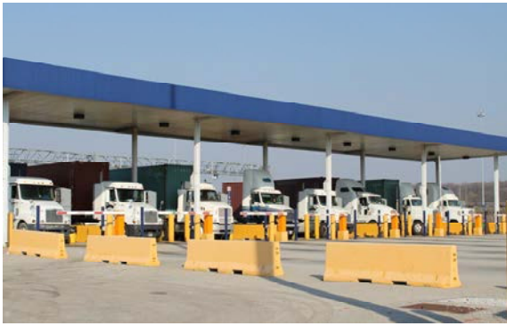
BNSF Multimodal Hub Automated Gate Control
