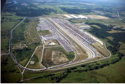
Aerial View of LPC Integrated Logistics Park/Multimodal Hub
