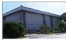
3 Kim Heng Warehouse 4 Penjuru Lane
