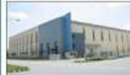
10 APC Distrihub 6 Changi North Way
