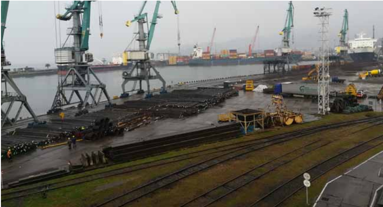
Batumi Port. Rail tracks for portal gantry cranes and rail tracks for rail wagons in close proximity to wharf and cargo working areas.
