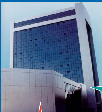
Central Office of SCC
