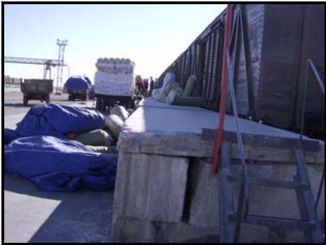
Platform Repairs/Expansion Station #1
