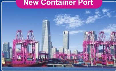
New Container Port
