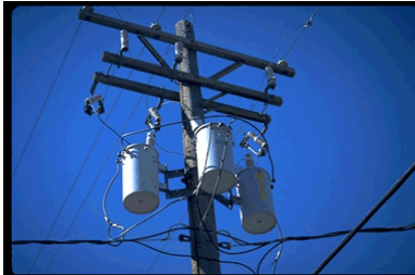
Rural Electric Cooperatives 119 (2,494 MW)
