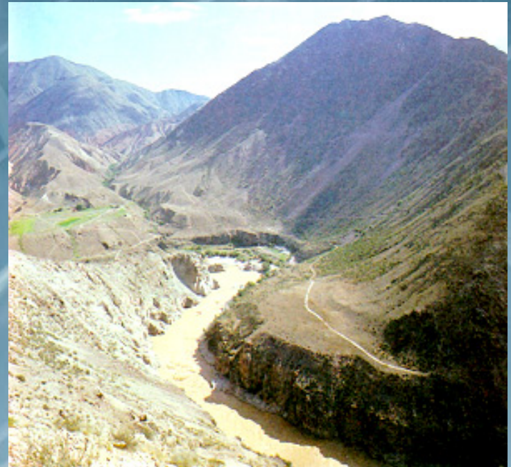
The HPP site according to the project
