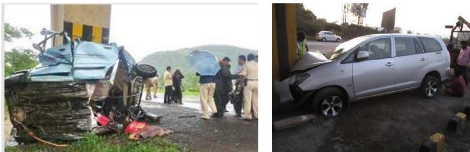
FIGURE 15: CRASHES ON THE EXPRESSWAY WITH OVERHEAD BRIDGE PILLARS.
