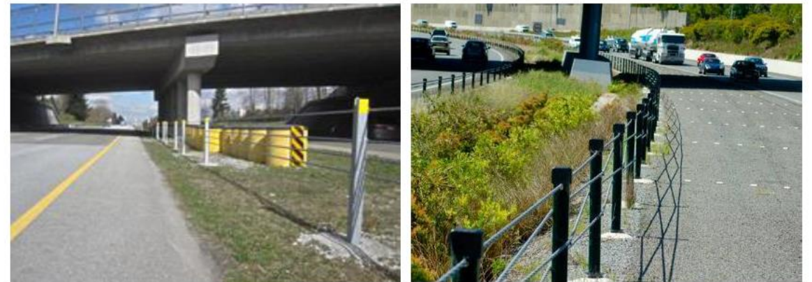
FIGURE 16: BRIDGE PILLARS GUARDED WITH IMPACT ATTENUATORS AND ROPE WIRE BARRIERS.
