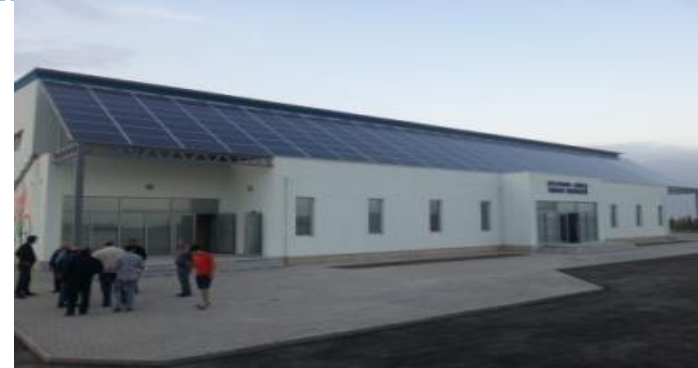
Sports Complex in Beylagan district (70 KW electric, 90 KW heating)
