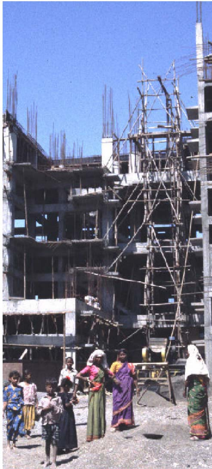
Photo 7 - The first Rajiv Indira rehabilitation block in progress
