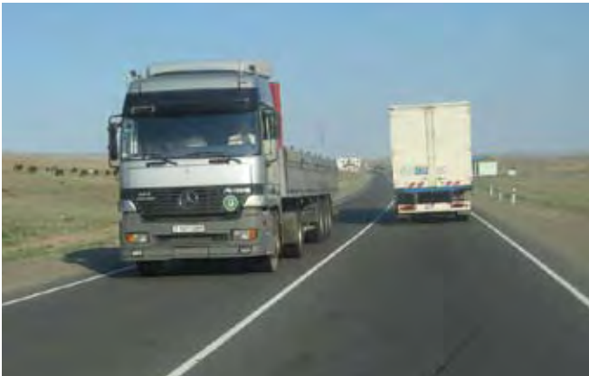
Almaty–Bishkek Road, Kazakhstan, CAREC Corridor 1b and Corridor 3
