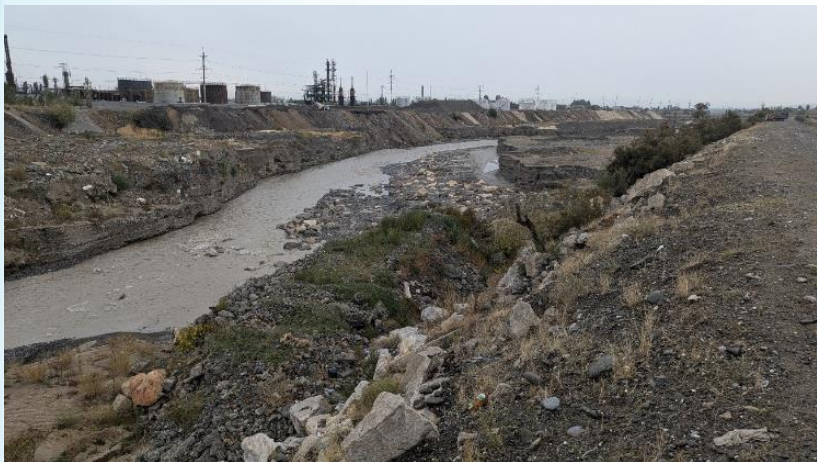
Erosion in Kugart river near Jalal-Abad. probably induced by upstream sediment extraction.
