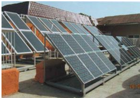
Heliosystem of hot water supply and 2 KW PV station in Fergana
