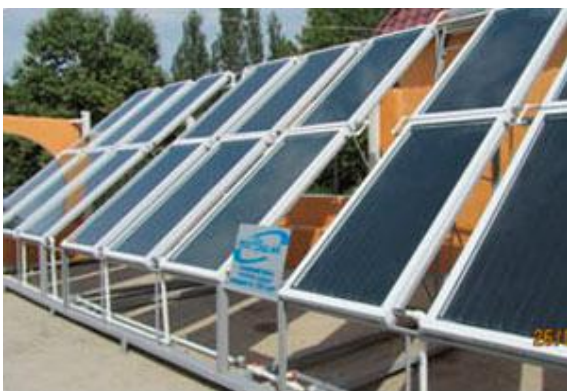
Heliosystem of hot water supply in Fergana
