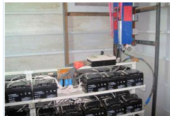
Energy storage system of 40 accumulators
