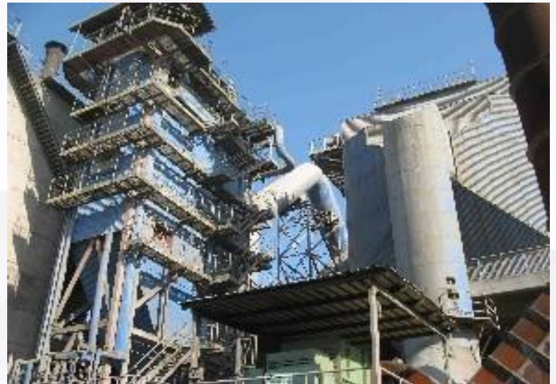
Power Generation of Waste heat
