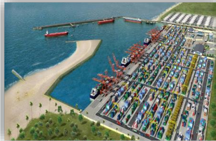
Construction of Anaklia Deep Sea Port
