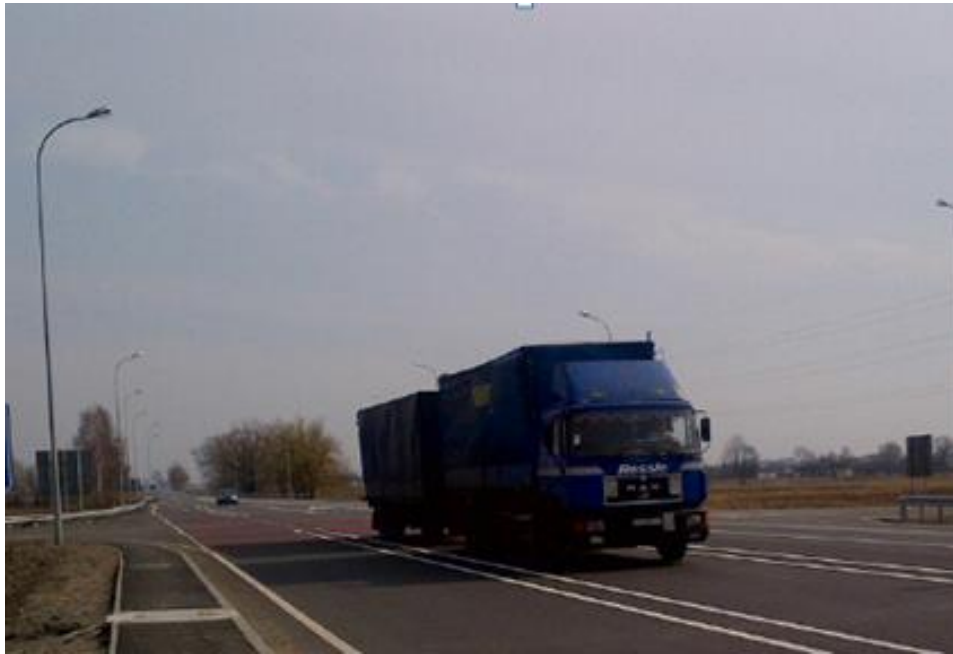
4-way junctions on high speed roads
