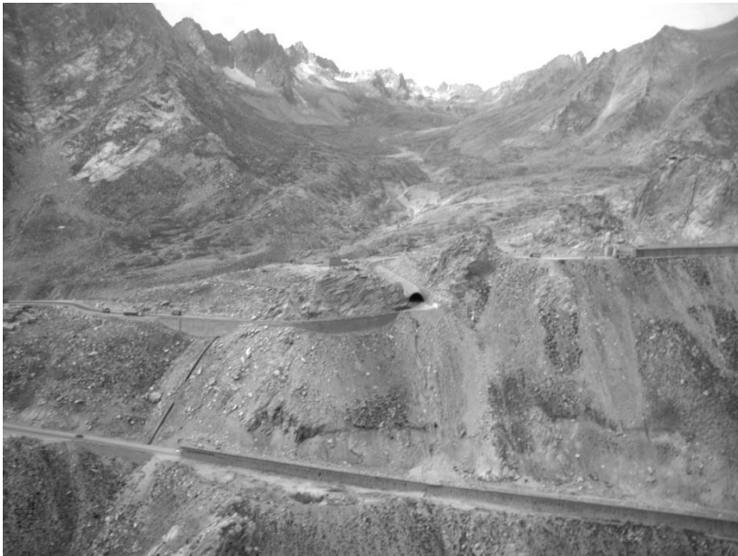
Salang Tunnel - South Portal, 2011
