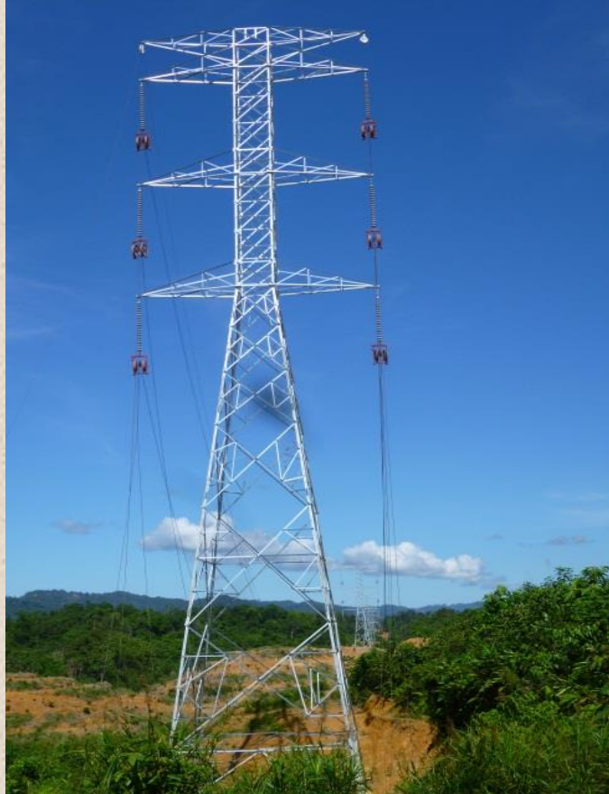
Hanging of running block and stringing pilot wire in the progress
