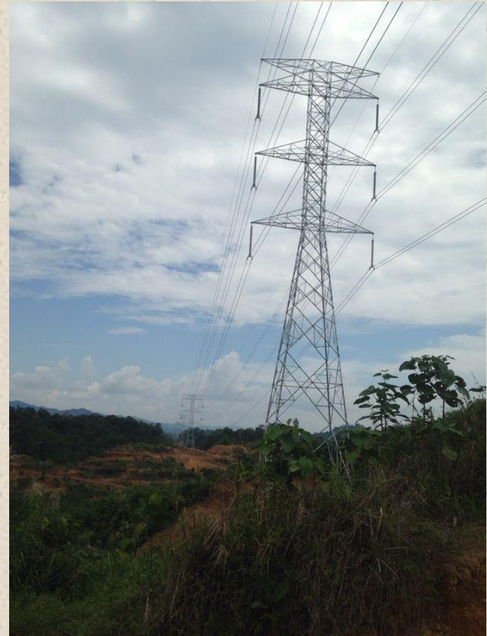
Overview of completed stringing and clamping work
