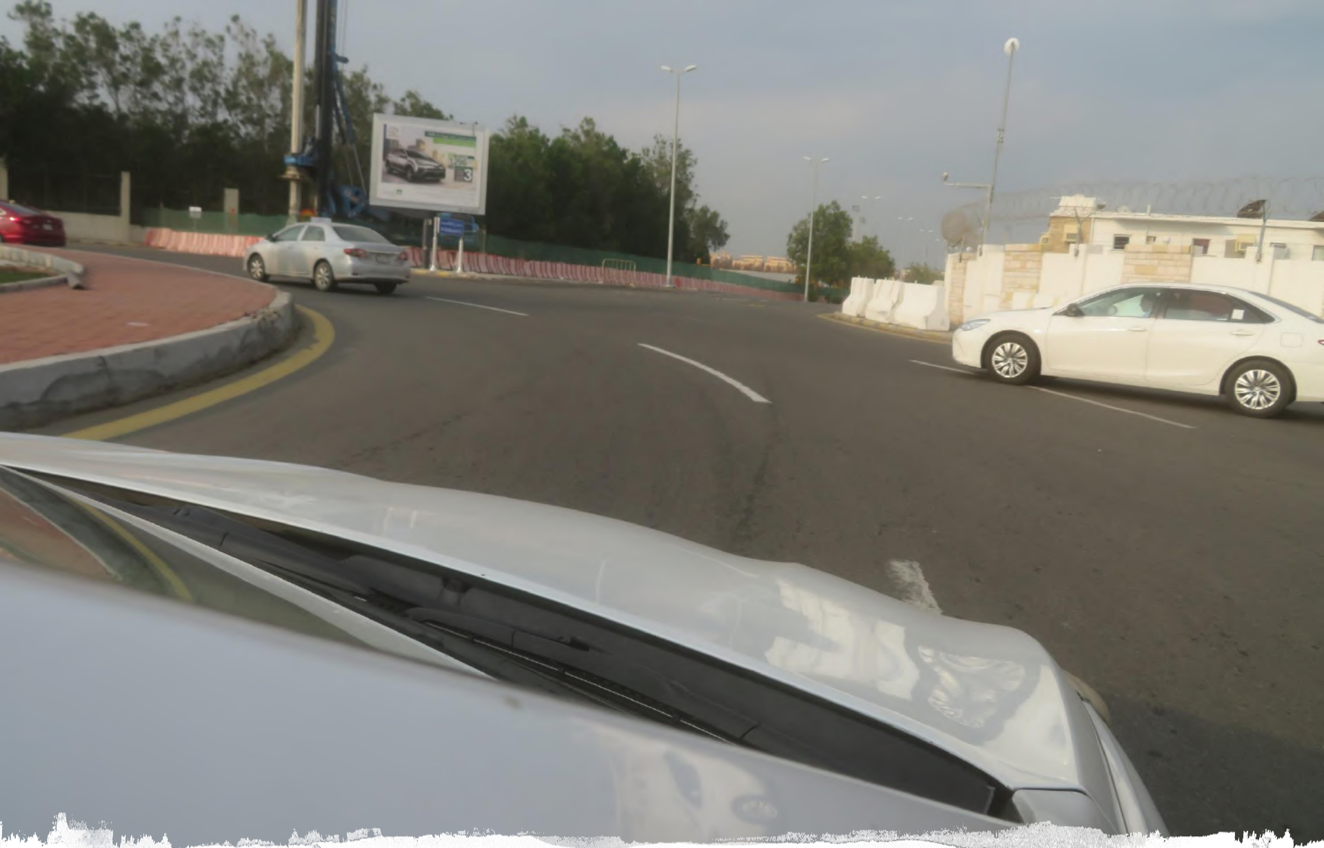
This multi-lane roundabout would benefit from “Exit” line marking
