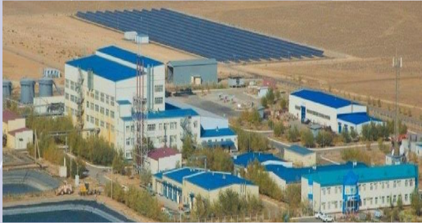
1 MW solar power station «DP Ortalyk» in South Kazakhstan Region
