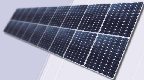
2 MW Solar Power station, Mangistau region
