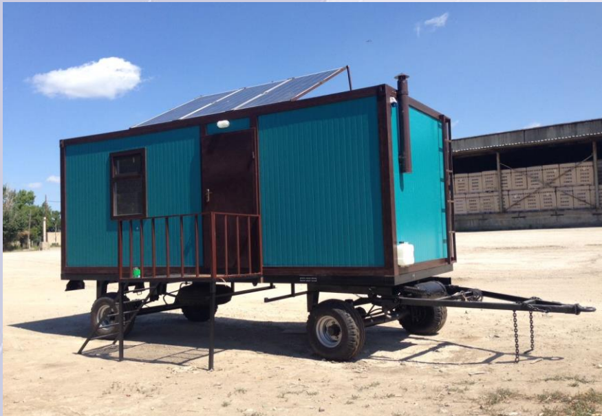
Mobile solar station 0.9 kW
