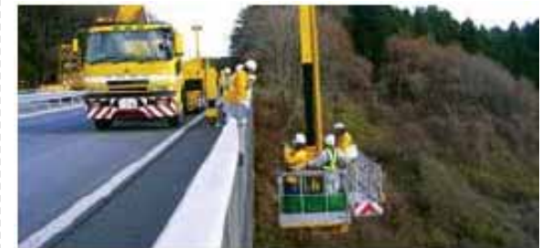
Daily/Periodical/Emergency inspection Bridge, Tunnel, Slope etc.
