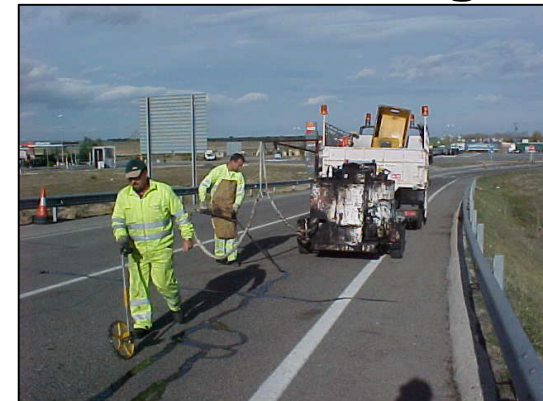
Cracks Sealing
