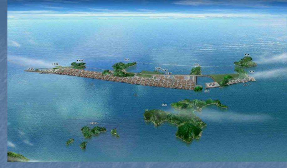
Phase III: Construction completed by the end of 2008. Added 7 more deep-water berths. Water depth: 17.5 meters. Port coastal line is longer, increased by 2600 meters. Designed annual handling capacity: over 9.5 million TEUs.
