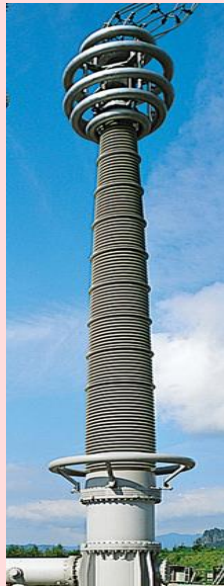
Gas Bushing for UHV Substation
