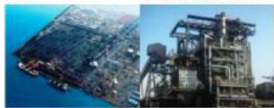
Nippon Coke & Engineering Co., Ltd. Kitakyushu Coking Works
