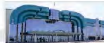
Multifunctional Building BCP-1 ICBC "Khorgos"
