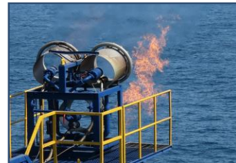
Flare from offshore production test
