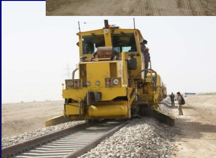
Track ballast stabilization and leveling
