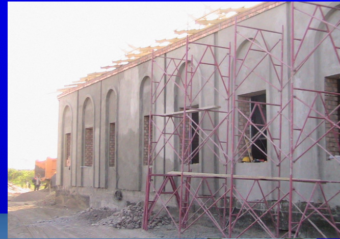
Stations being built
